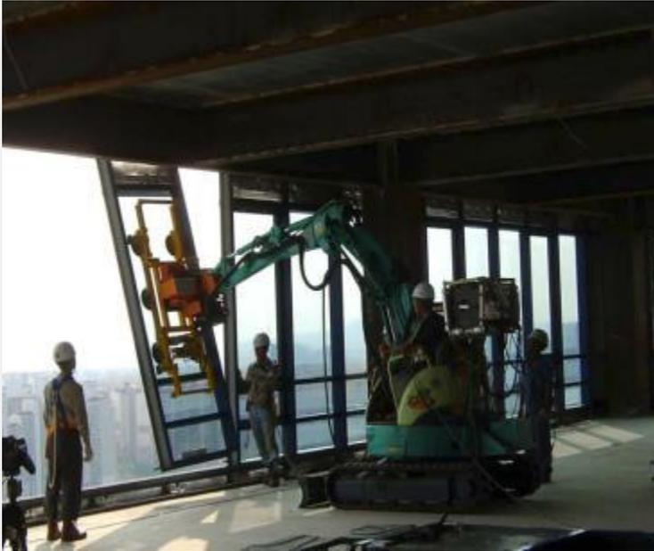
ASCI (Automation System for Curtain-wall Installation)
